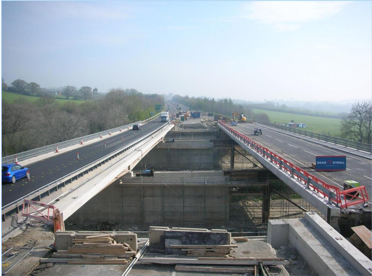
Bridge slide procedure minimises traffic disruption on one of Devon’s busiest roads. Leading controlled hydraulic movement specialists Bill Boley Ltd have completed a complex bridge sliding project on the A30 in Devon for contractors Dean & Dyball.
