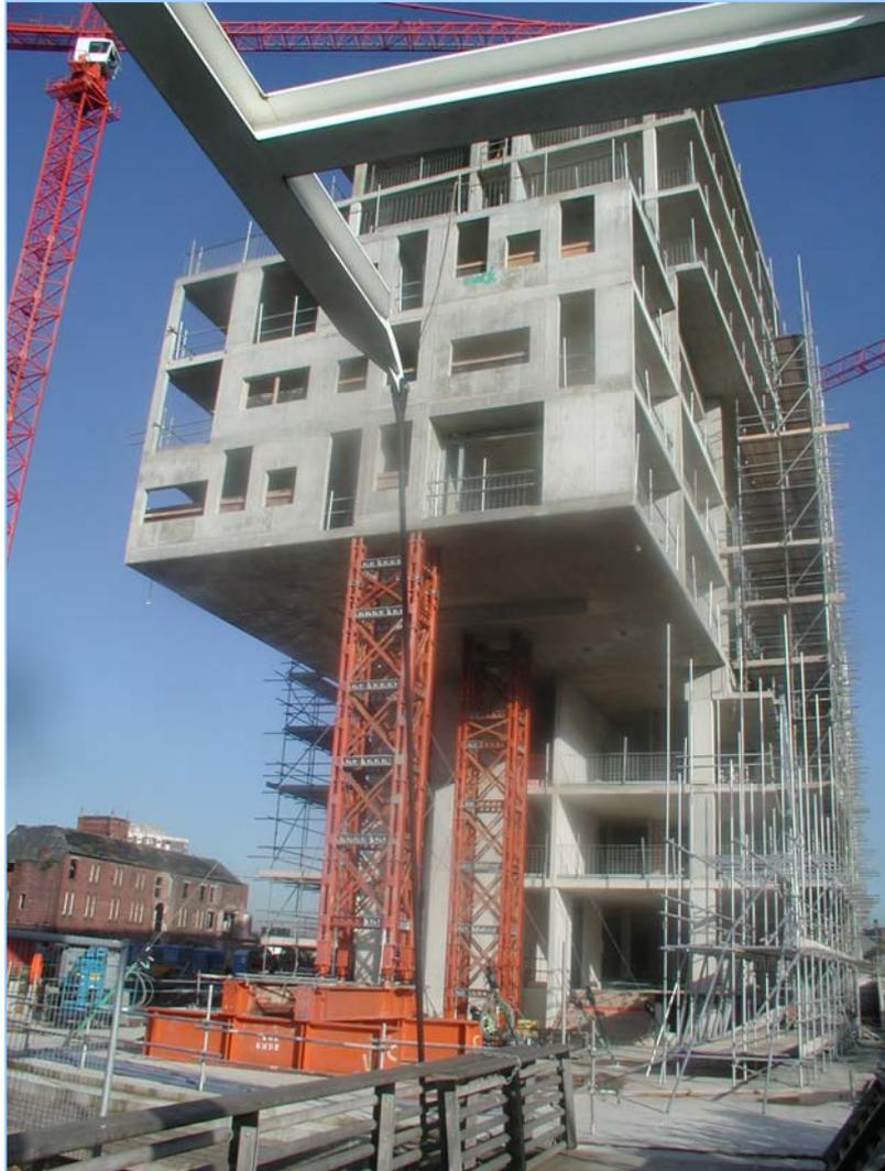
Hydraulic movement specialists Bill Boley Ltd have successfully completed a vital jacking and load measuring project during the construction of the so-called Chips building on the New Islington Millennium Village site in East Manchester.
