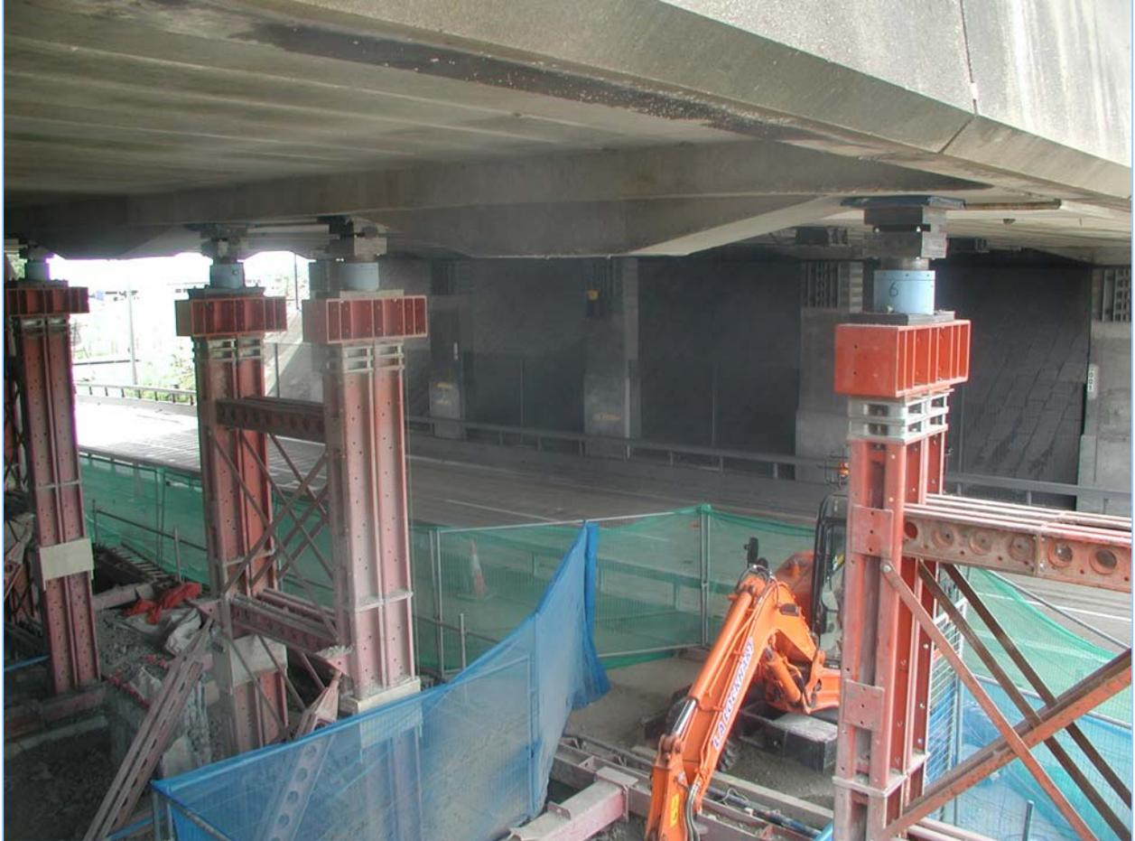
Hydraulic movement specialists Bill Boley Ltd have completed a complex £750K jacking and load measuring project during major refurbishment work at junction 13 on the M4 in Berkshire, adjacent to Chieveley Services.
