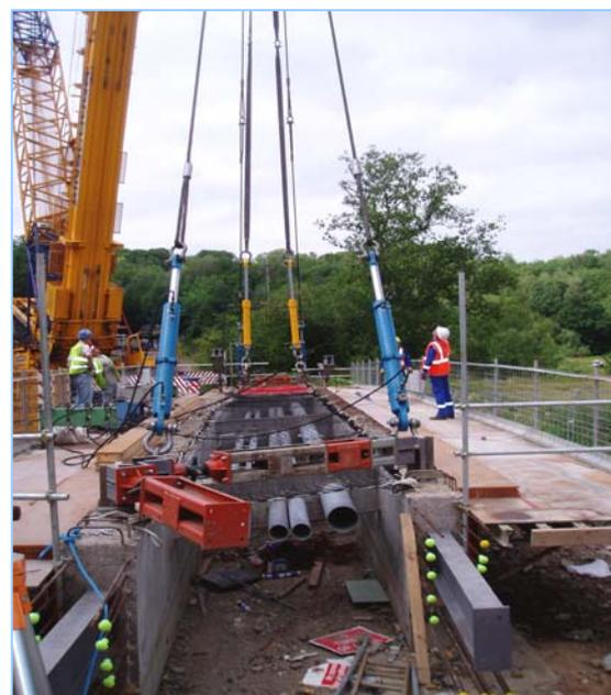
Lifting the middle section into place between to the two abutments presented a number of challenges. Although the section only weighed around 80 tonnes, the combination of
