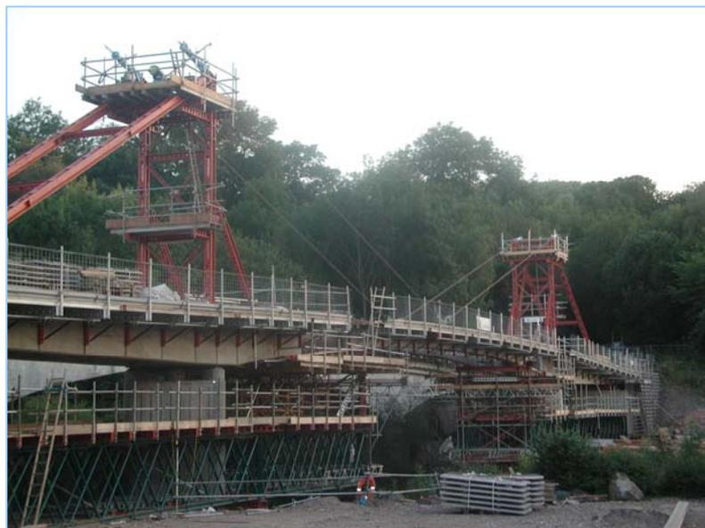
unison to apply the required pre-determined upward force of 470 kN. This arrangement, with the cables tensioned, remained until August 2006 when the concreting the infill had been completed and sufficiently cured.
