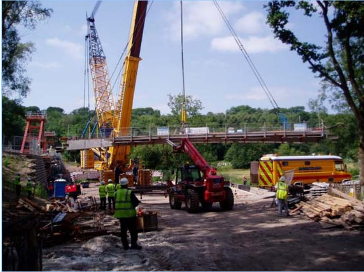
surrounding vegetation and the distance it needed to be lifted required the use of a massive 1000 tonne mobile crane operated at full stretch. In order to ensure the section was lifted evenly, Bill Boley installed six special hydraulic cylinders, one at each lifting point at the ends and centre. By combining the readings from the LVDTs and the hydraulic pressures from the
