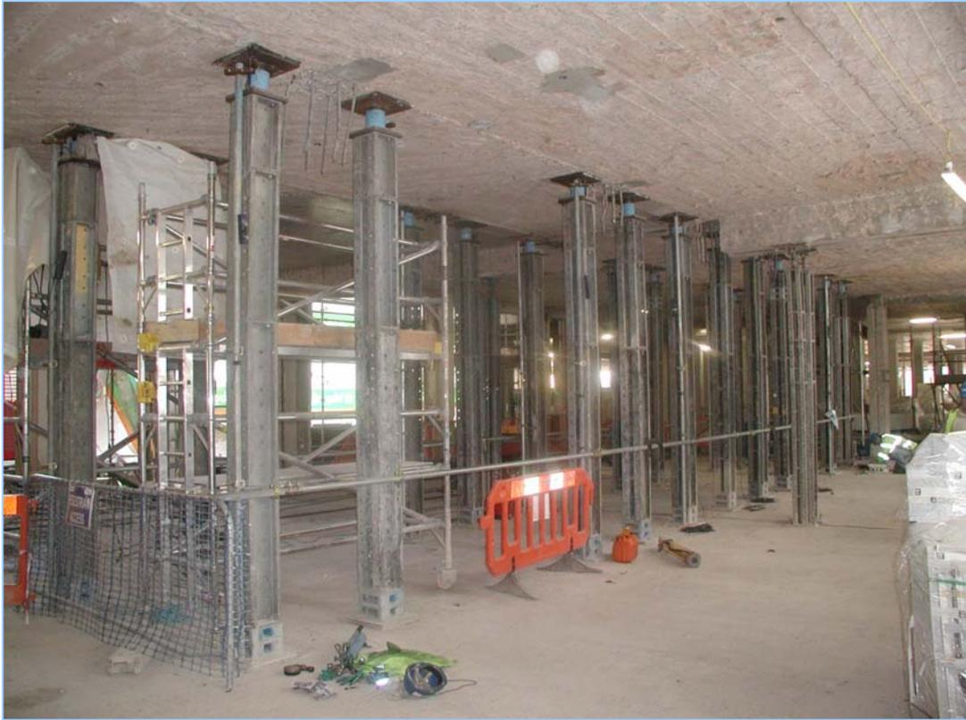
Complex jacking procedure ensures building structural integrity is maintained
